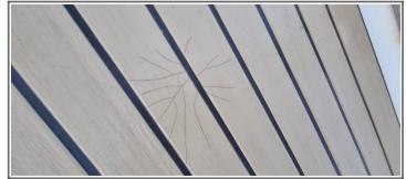
integrity of these components. However, a minimal number of small star crazes were observed on the foredeck. It is important to note that these crazes were of a non-structural nature and, as such, do not pose a significant concern regarding the vessel's overall safety and durability.
